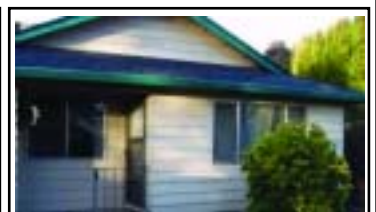
YAMHILL COUNTY HOME IN QUIET CUL-D-SAC. 3 bed, 1.1 bath, 1074 sqft Newberg home with newer roof and sprinkler system plus floor allowance and 1 year warranty. $210,000
